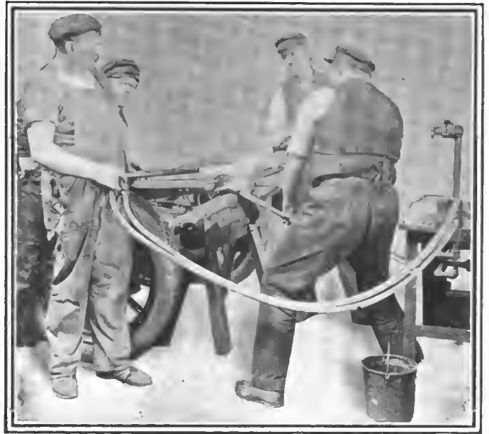
Executing an autogenous-welding job on an automobile. Two men handle a flame each and another assists
